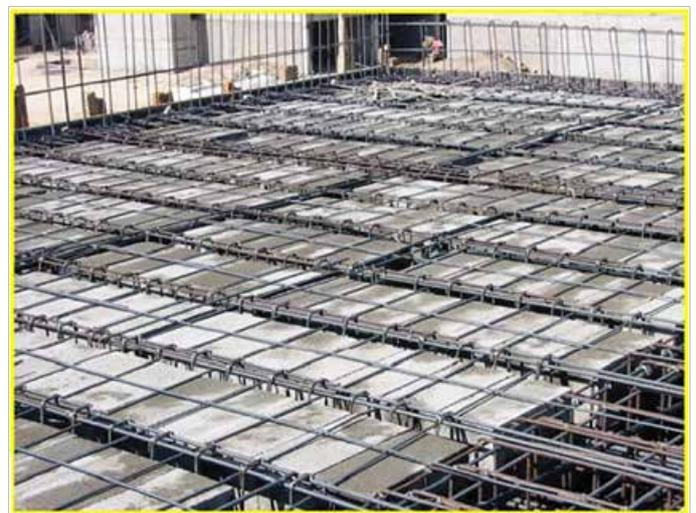
Fig 2: One-way hollow slab arrangement (sources: (Hosny, 2008)
